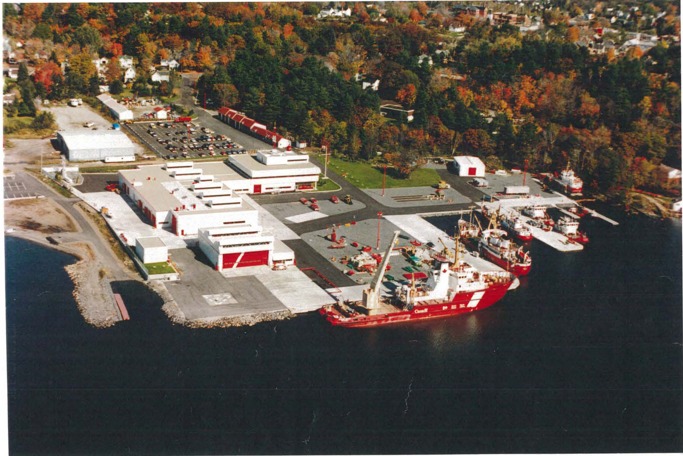
COAST GUARD FACILITY
