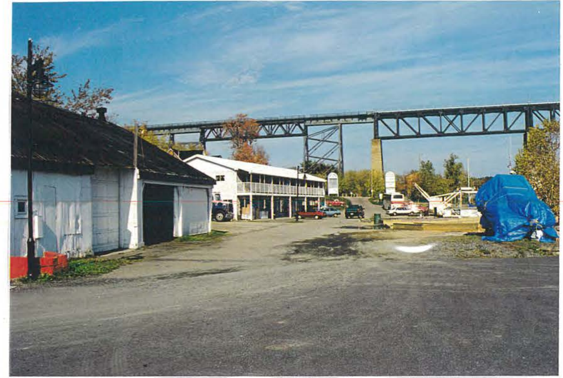
2. View north along west side of Seguin River
